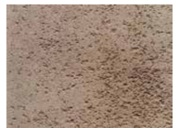
Condition D Blasted to Sa2.5
