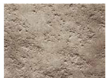
Condition D Blasted to Sa3
