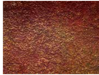
Condition C Unblasted
