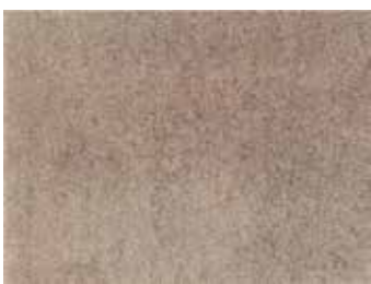
Condition A Blasted to Sa2.5
