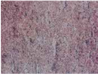
Condition A Blasted to Sa1
